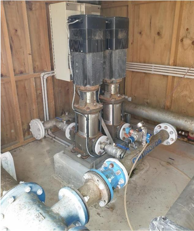
Figure 19: Reticulation Booster Pump Skid
