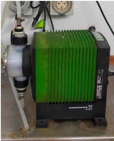
Figure 13: Alum Dosing Pump
