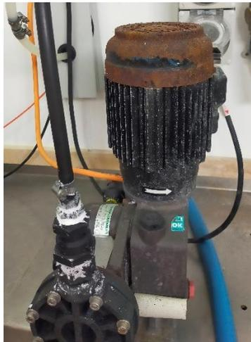
Figure 14: Soda Ash Dosing Pump
