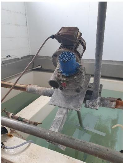
Figure 3: Alum Batch Tanks
