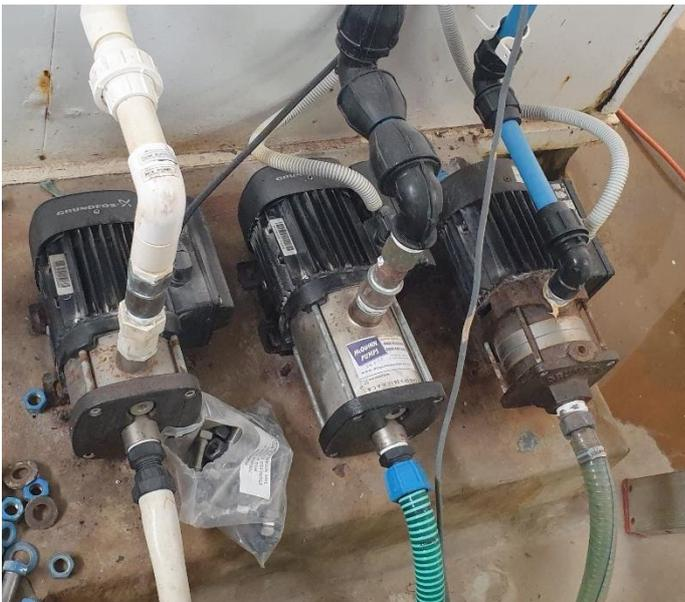
Figure 16: Chemical Carrier Pumps
