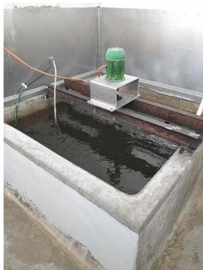
Figure 4: Soda Ash Batch Tank
