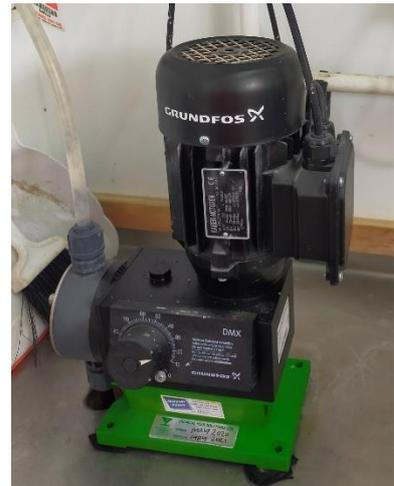
Figure 15: Polyelectrolyte Dosing Pump
