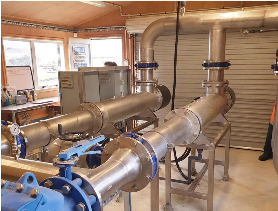
Figure 8: Duty/Standby UV Reactors
