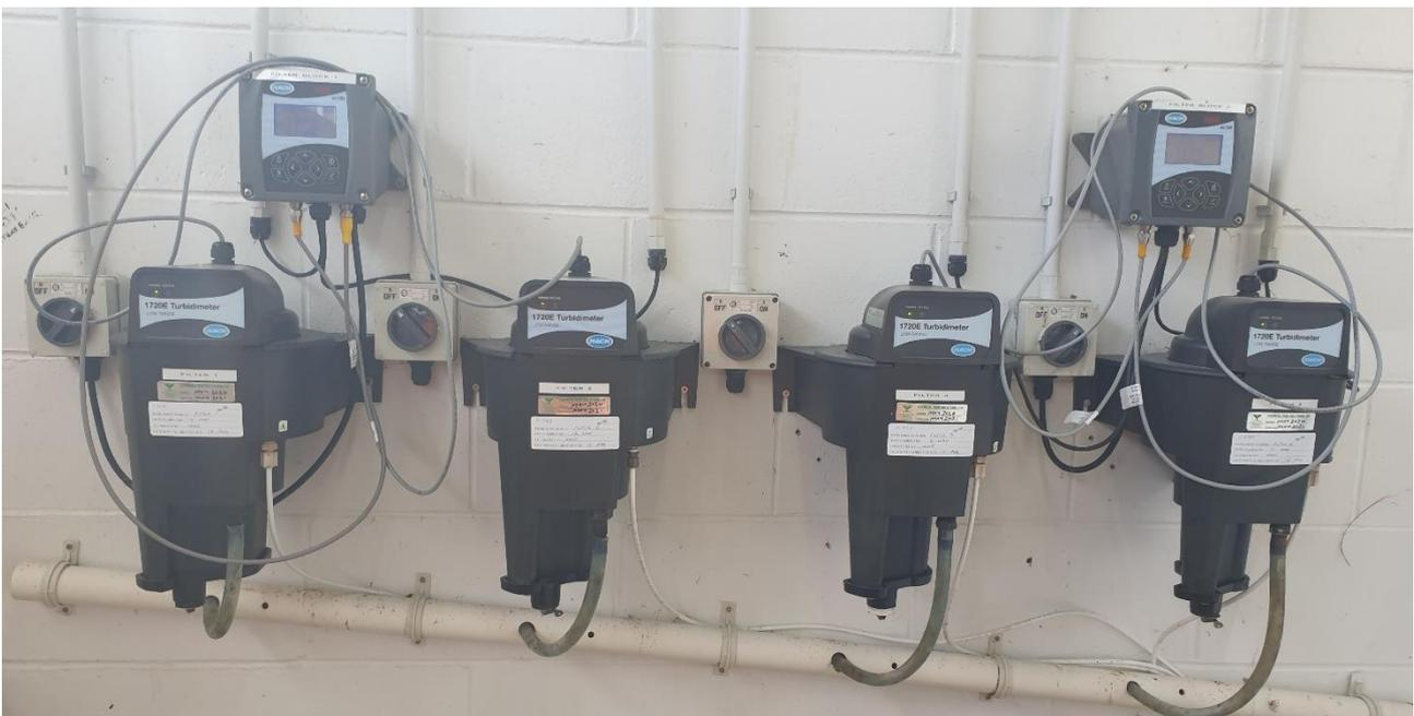
Figure 18: Turbidity Analysers and Transmitters for Filters
