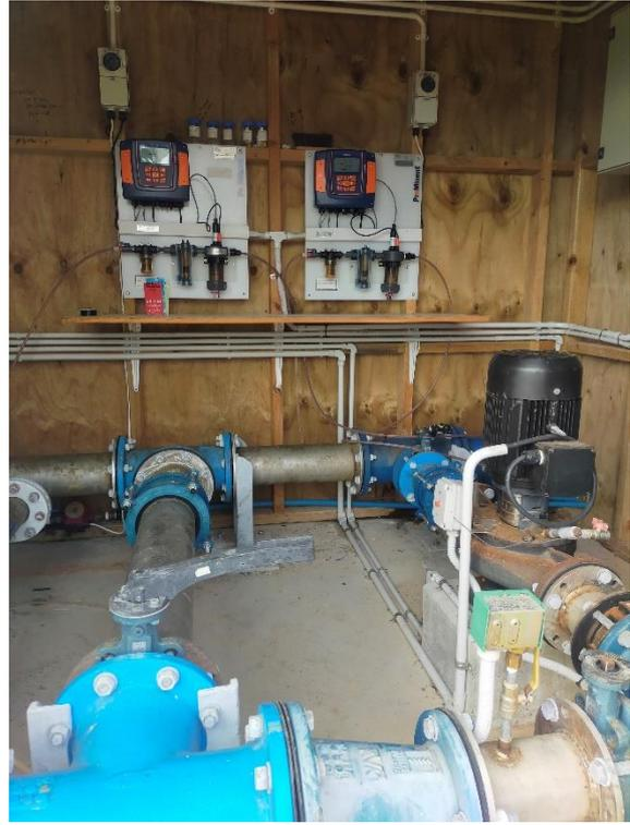
Figure 20: Final FAC and pH Analysers
